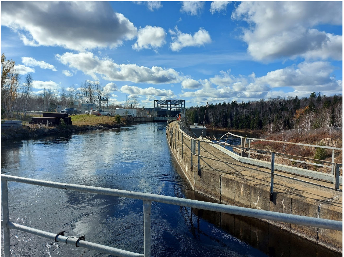
Figure 2-4 Stinson Intake Canal
