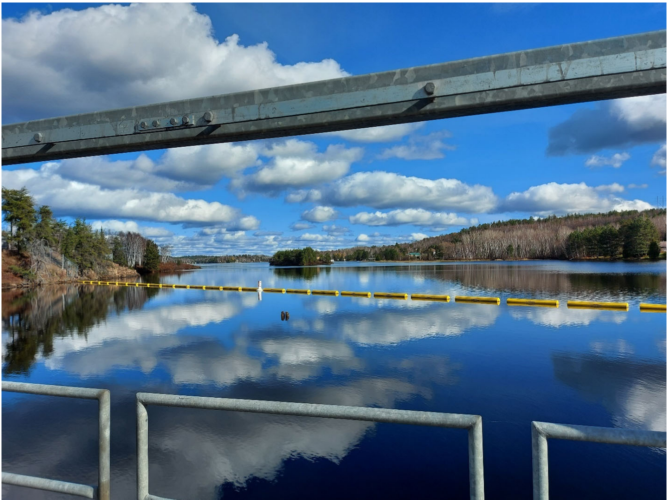
Figure 2-3 Stinson Reservoir (looking upstream from the main dam)
