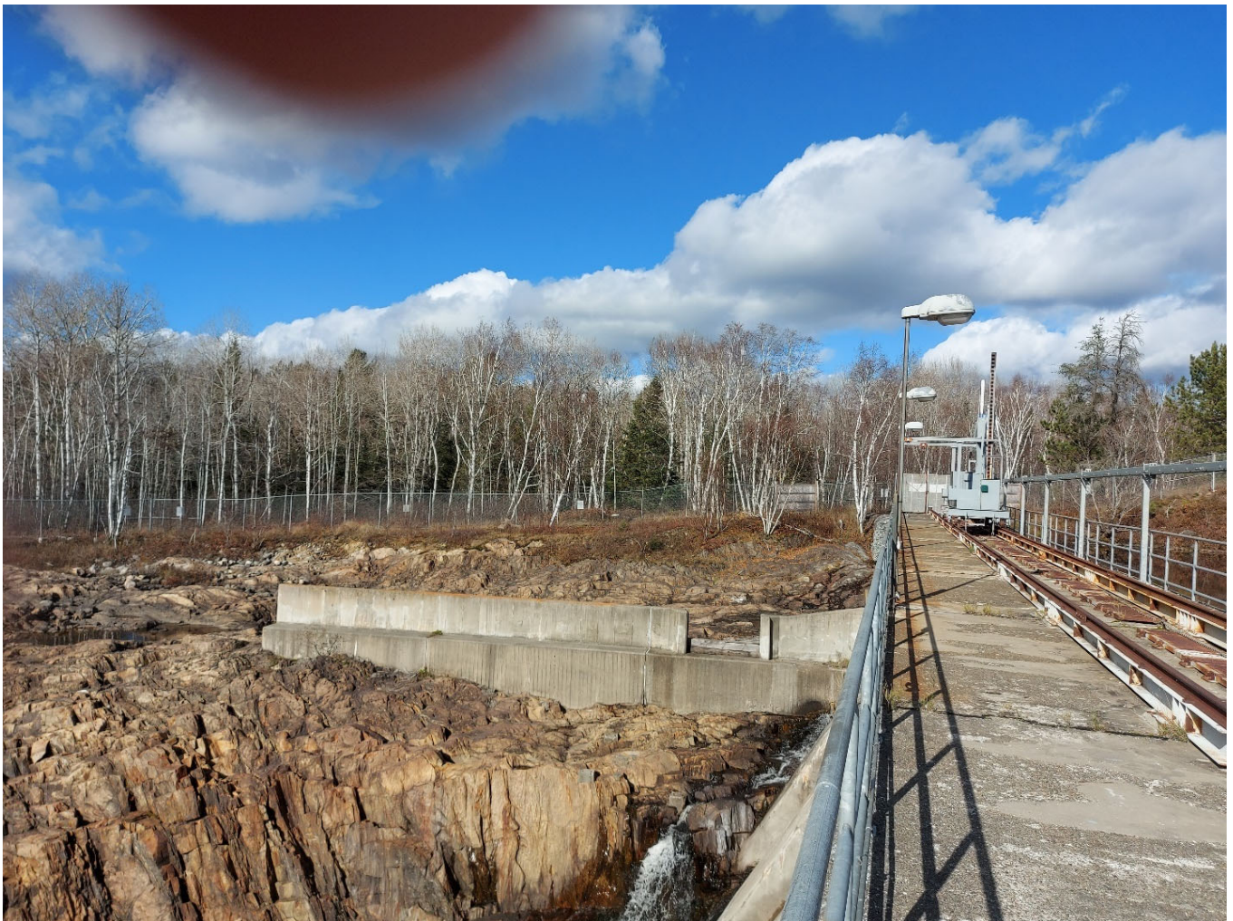
Figure 2-5 Stinson Main Dam
