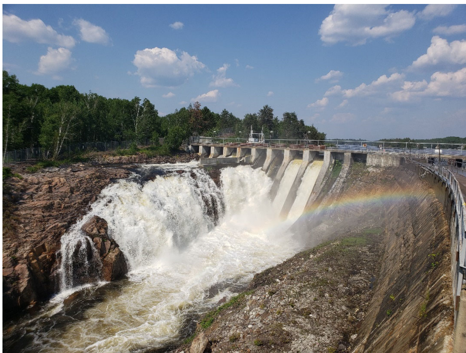
Figure 2-7 Stinson Spillway (likely 43.8 cms showing for the day)
