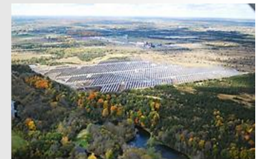
SunEdison Canada First Light Solar Energy Park
