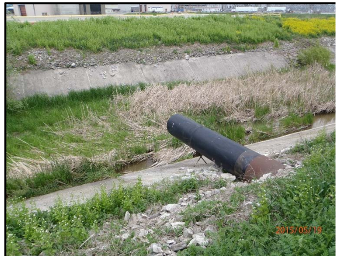
Photo 8. WC8 – OPG Coal Pile and Drainage Ditch- May 2015
