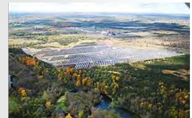
SunEdison Canada First Light Solar Energy Park
