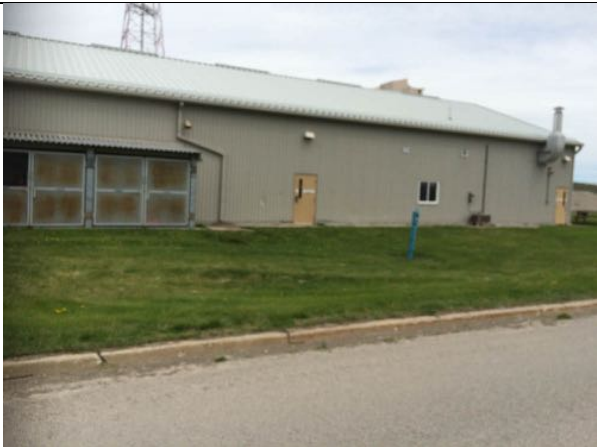
Plate 1: Disturbance via grading and utilities around western outbuilding.
