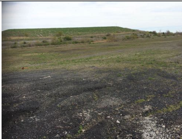
Plate 2: Coal yard facing north east showing ash storage mound and extensive grading.
