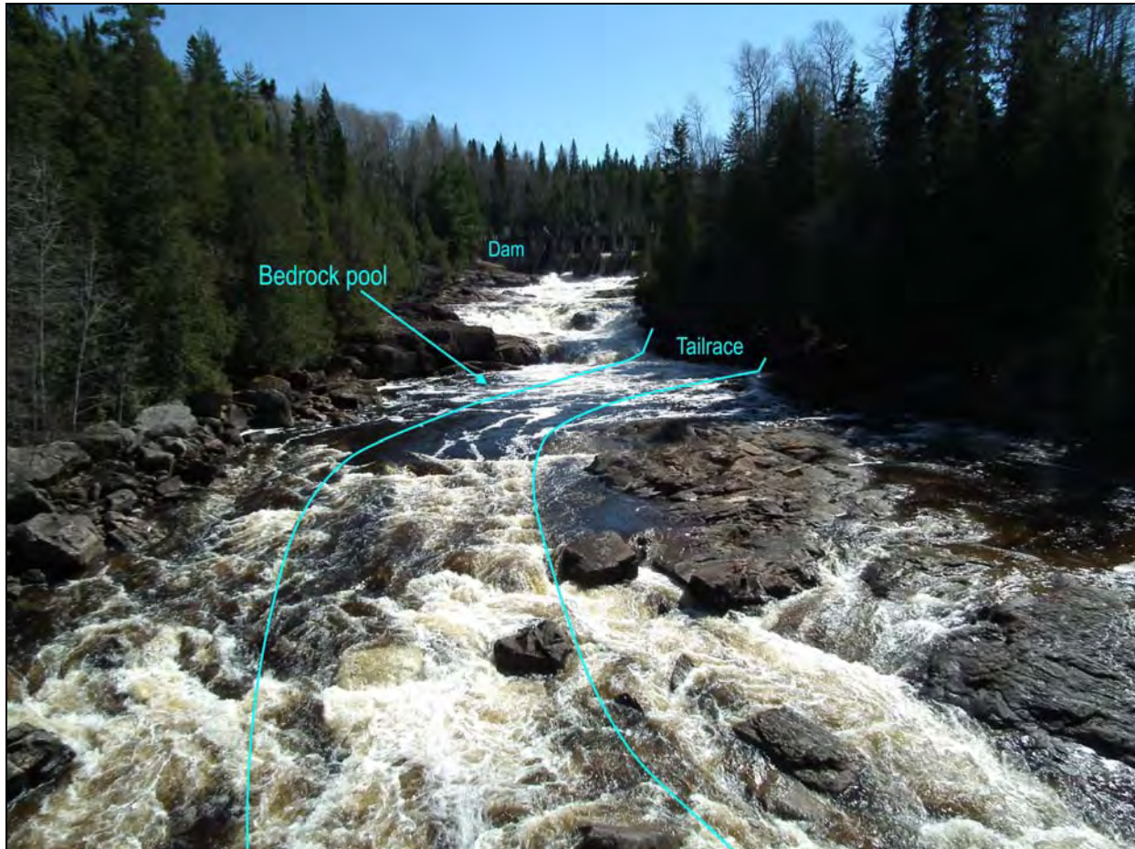
Photograph 3-4 View Upstream from the Road Bridge, May 8, 2011. The Approximate Location of the Proposed Tailrace Channel is Shown
