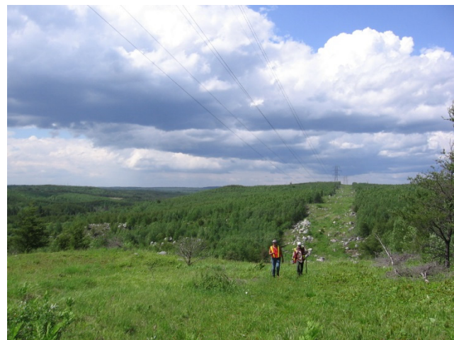
Existing 115 kV Hydro One Transmission Line
