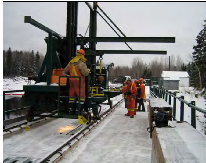
Water control at the dam
