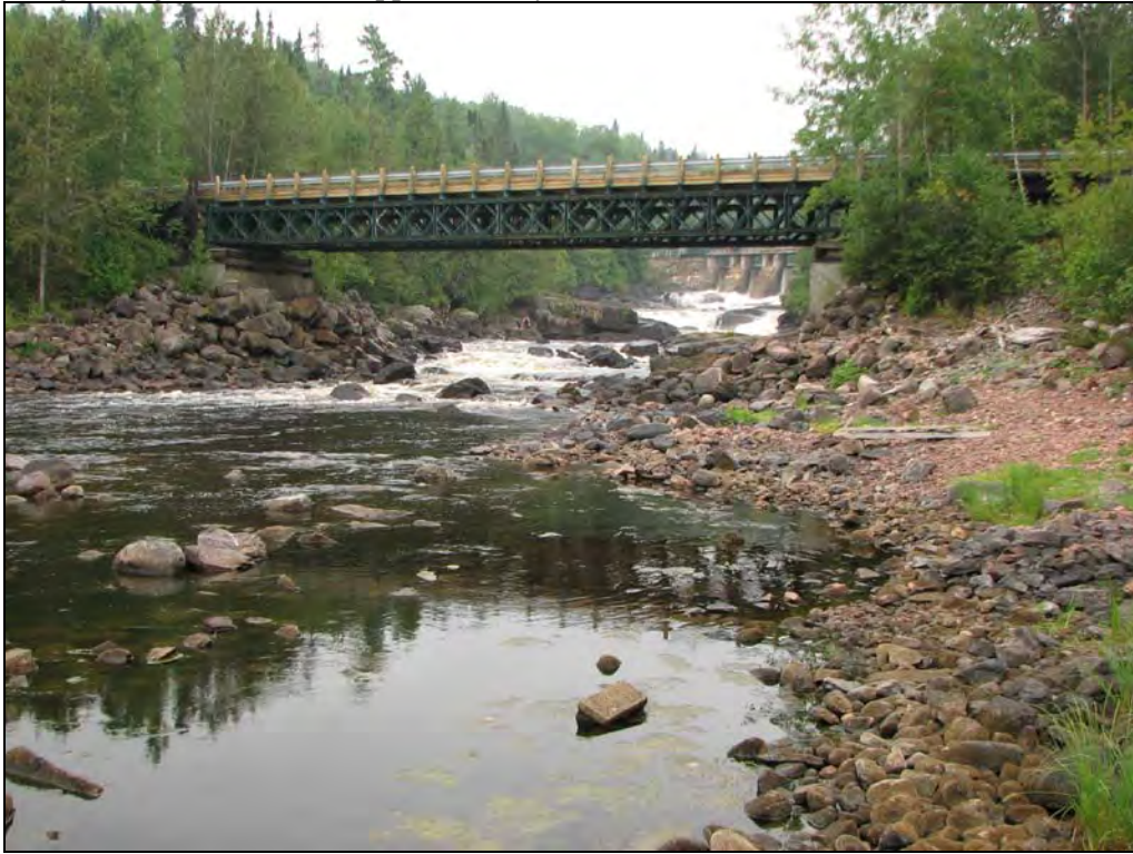
Photograph 6. View upstream along shallow west side of the pool located downstream of the road bridge. August 28, 2007. Approximately 7 \text{ m}^3/\text{s} .
