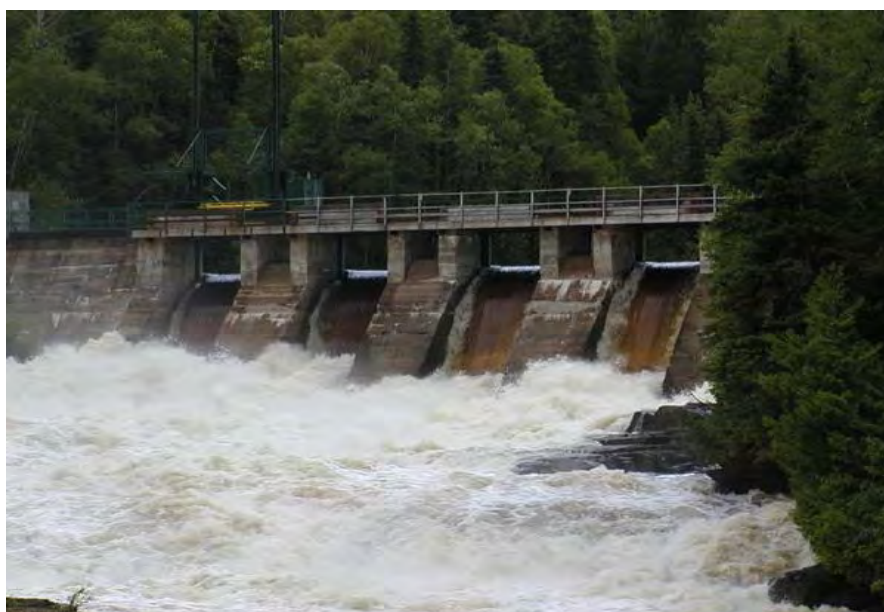
Photograph 2-1 Mattagami Lake Control Dam
