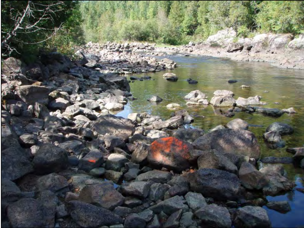
Photograph 4-3. 2.5 m 3 /s. Upstream view at approximately 150 m downstream from the road bridge.
