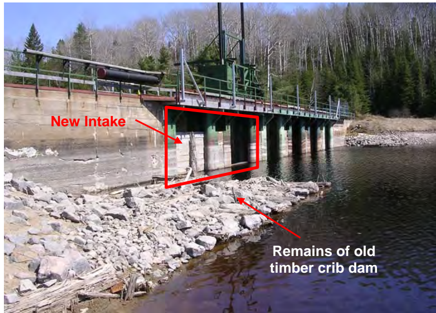
Photograph 2-7 Dam and Intake Structure
