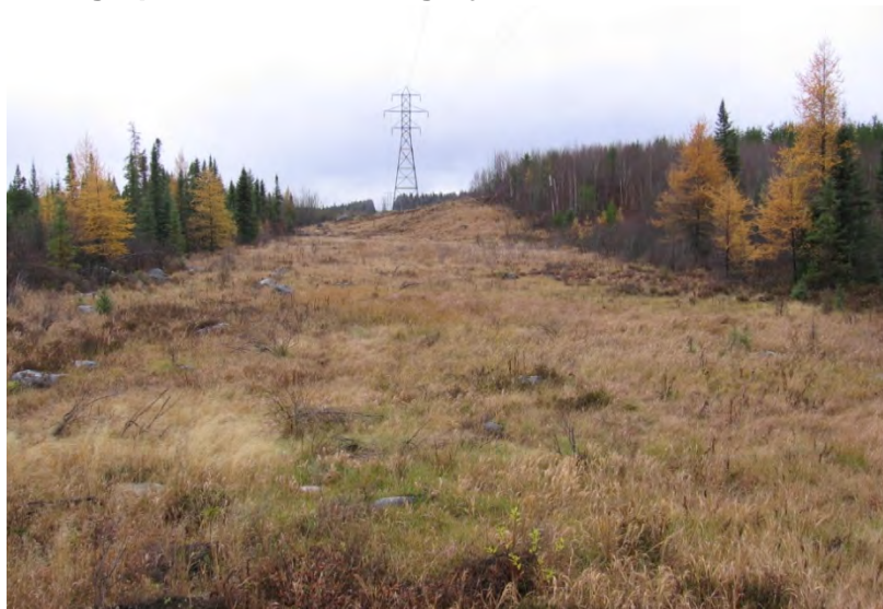
Photograph 2-13 Existing Hydro One Transmission Line
