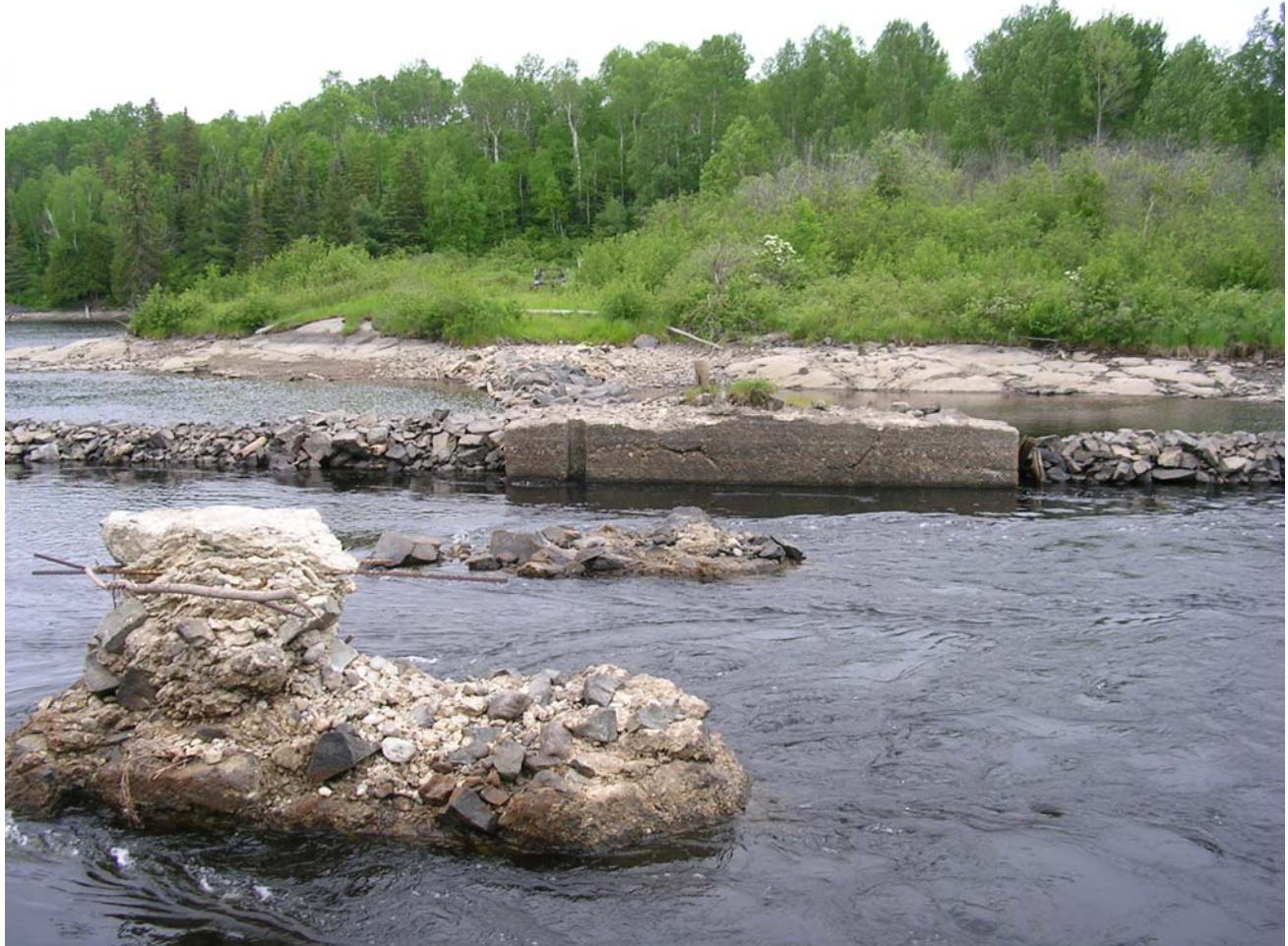
Photograph 1.2: Existing Submerged Structure at Low Water Levels, Hound Chute GS Forebay Inlet
