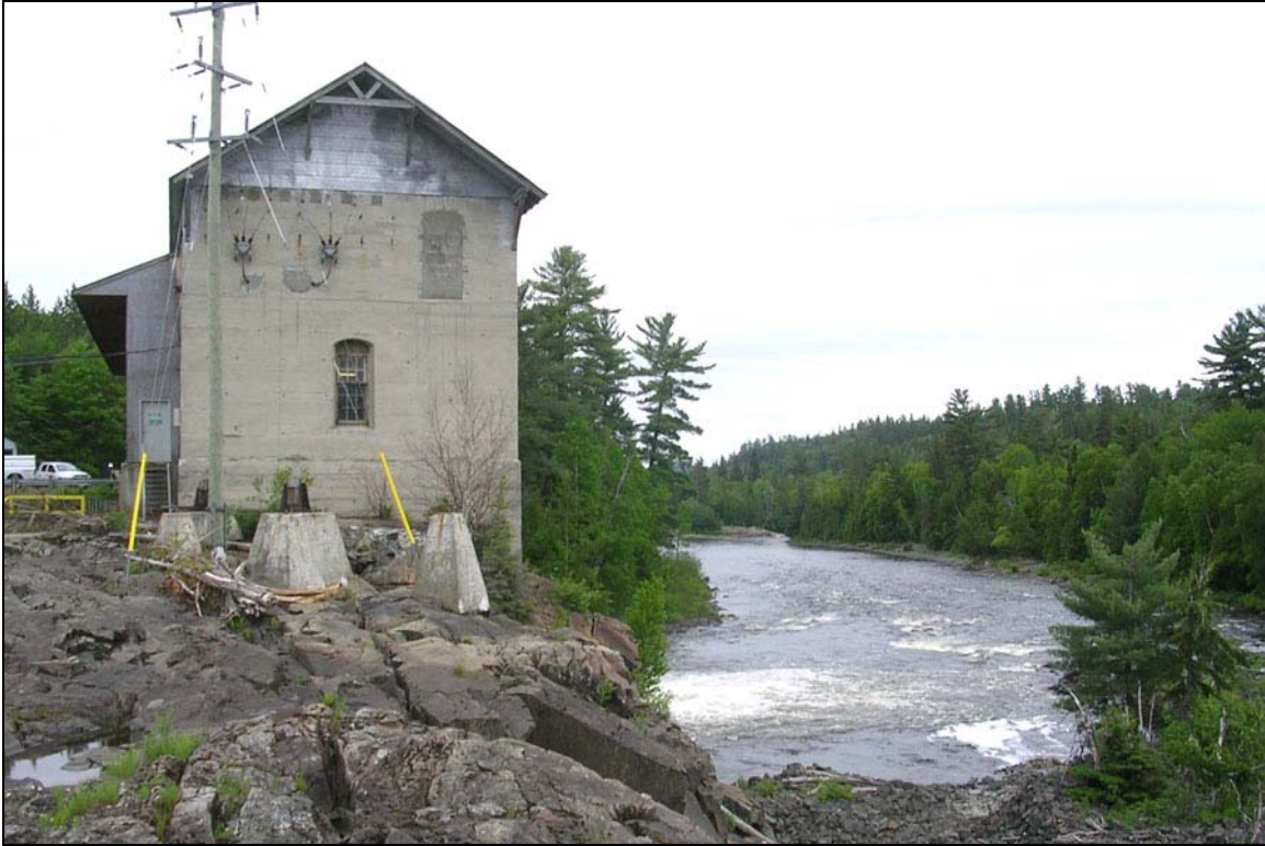
North gable end of the powerhouse with the transmission line.
