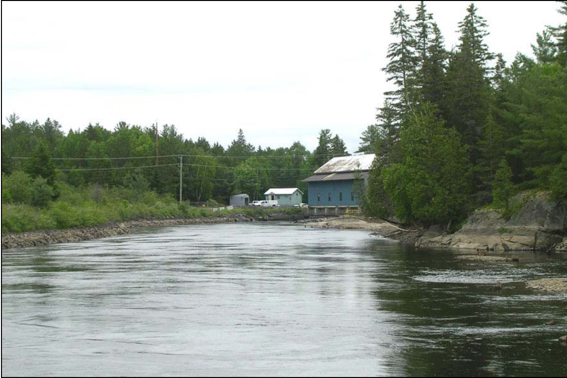
View south along the canal to the powerhouse.
