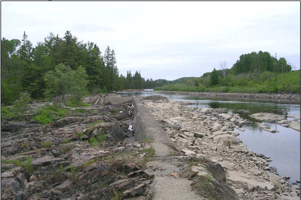
View north along the canal to the headrace intake.
