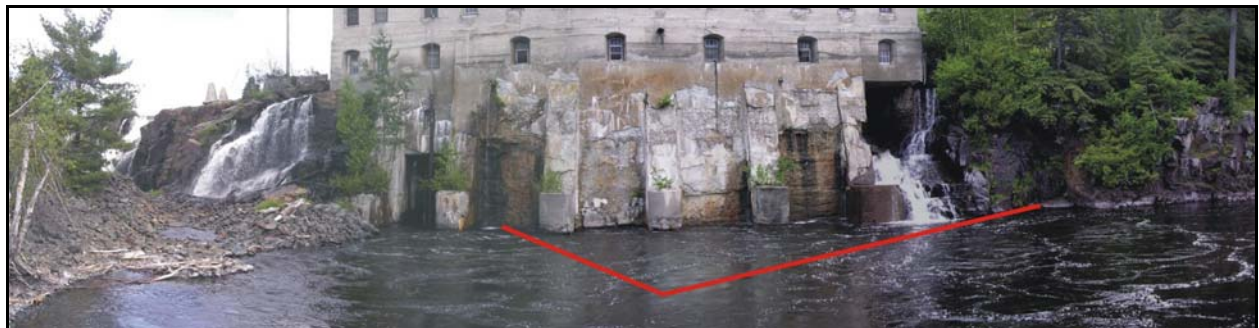
Photograph 3.3: View of the Hound Chute GS Tailrace. (Note: red line shows approximate downstream location of proposed GS.)
