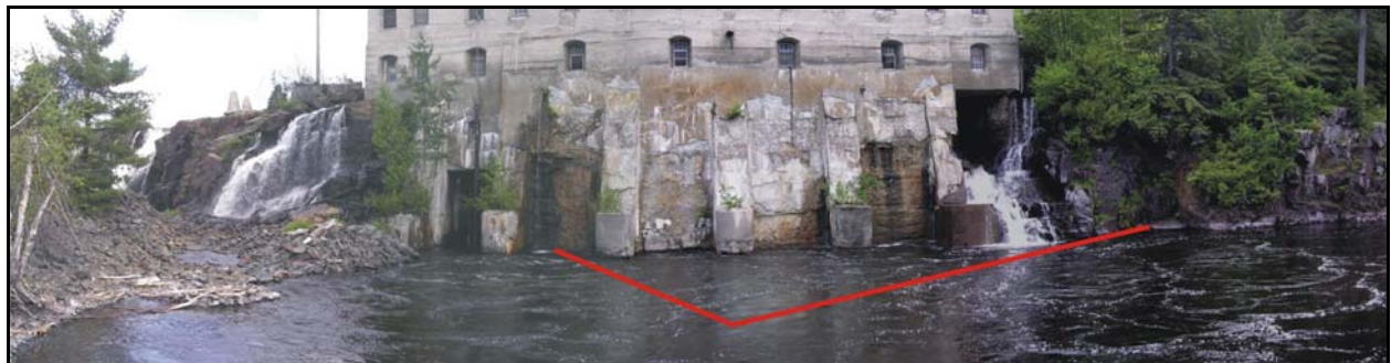
Photograph 2: Tailrace of existing GS. June 20, 2006. Red line shows approximate downstream location of proposed GS.
