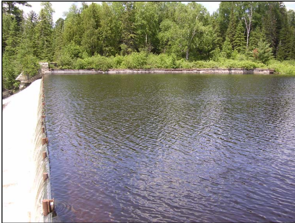
Photograph 3.4: View of Upstream Side of the Crest Weir at the Upstream End of the Spill Channel.
