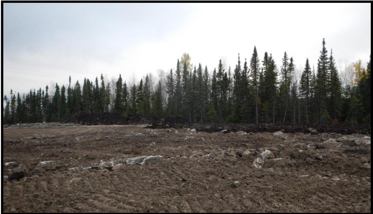
Figure 1: Little Long sediment pond topsoil stockpile
