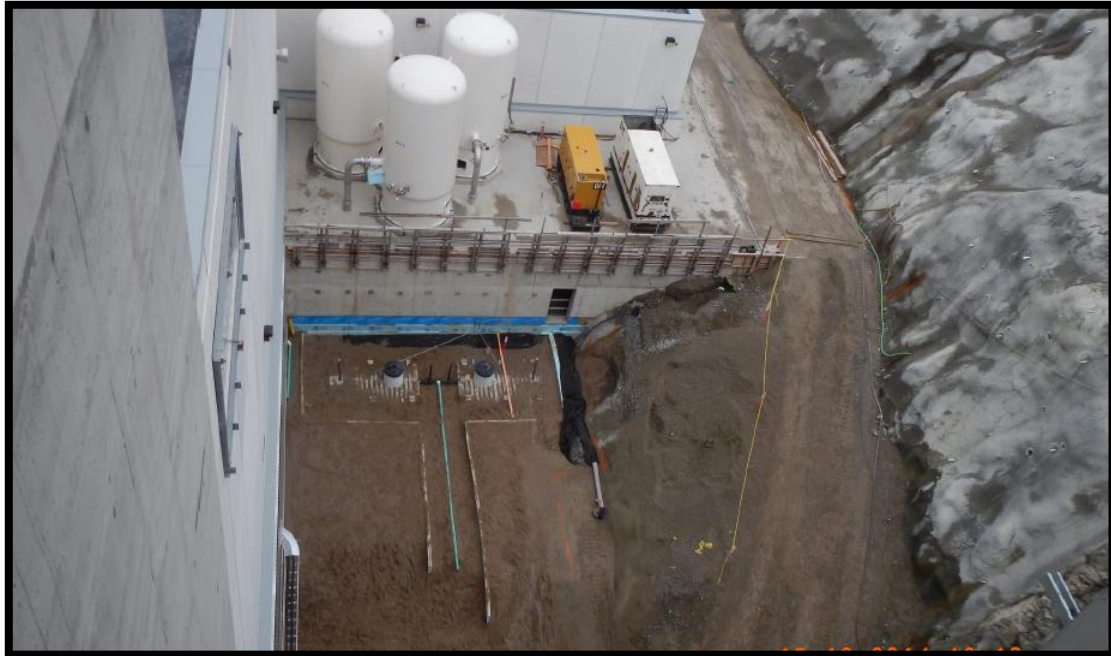
Figure 4: Smoky Falls Sewage Holding tank installation
