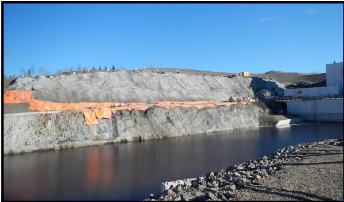
Figure 5: Smoky Falls Shotcrete application
