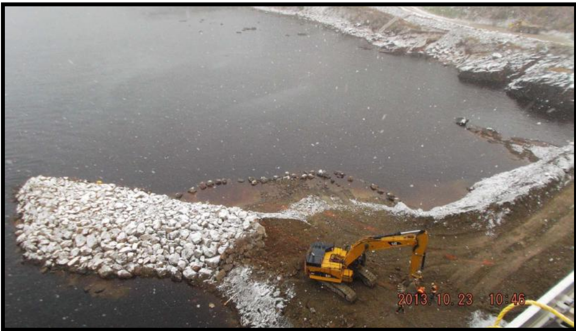
Figure 2: Harmon Marine Pad removal
