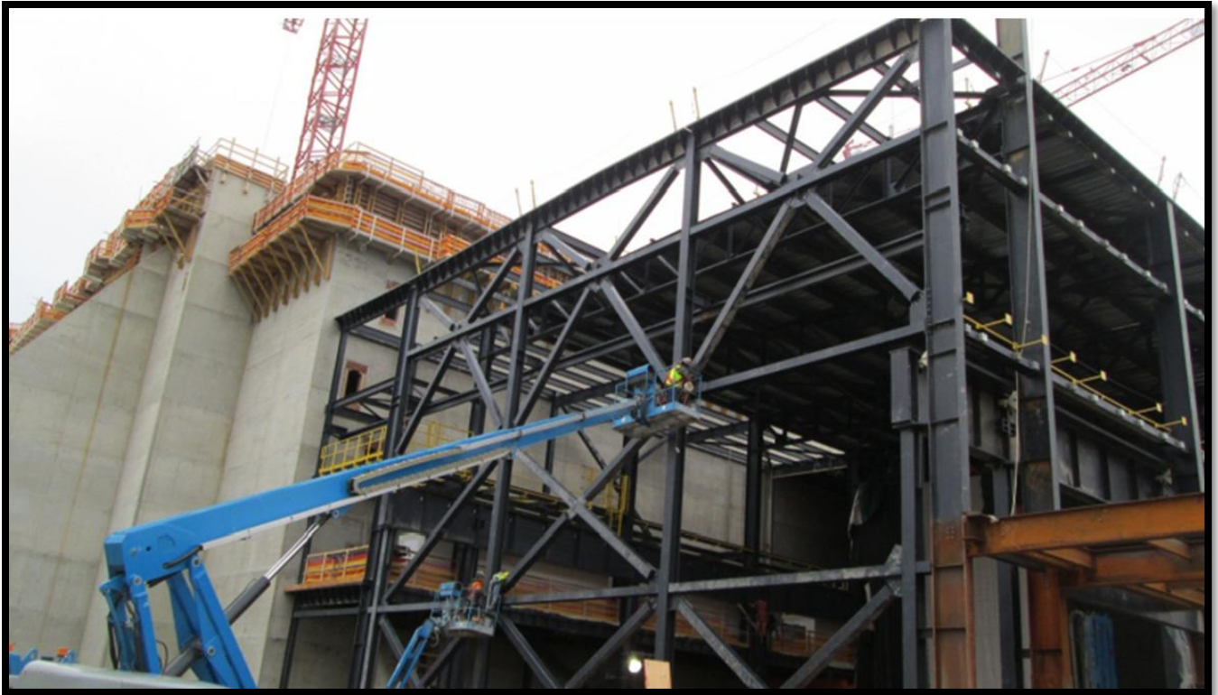
Figure 4: Smoky Falls – Superstructure erection
