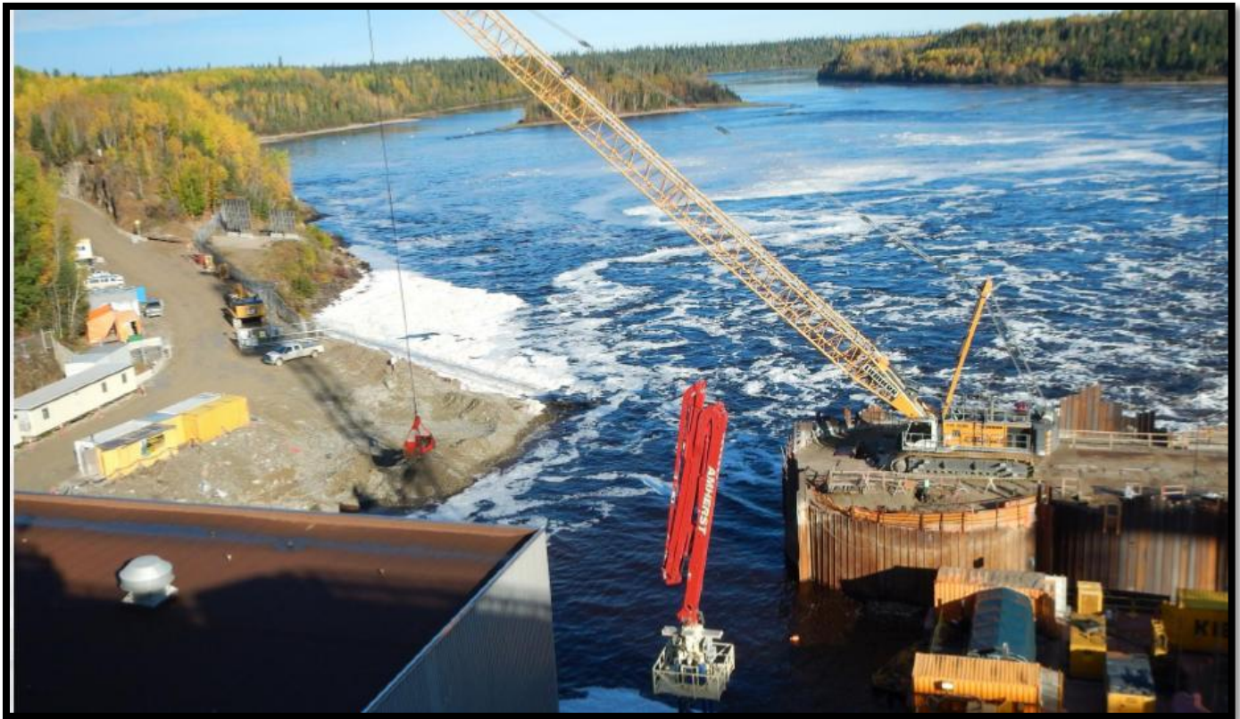
Figure 3: Kipling – Earth berm removal
