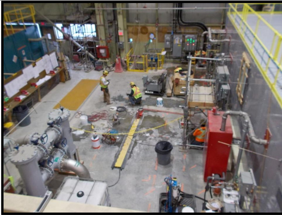
Figure 3: KAP grouting crew working on concrete at west of Kipling unit 3.
