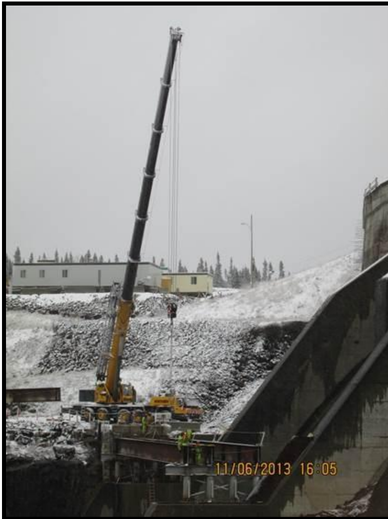
Figure 2: Harmon Bridge Dismantling.jpg
