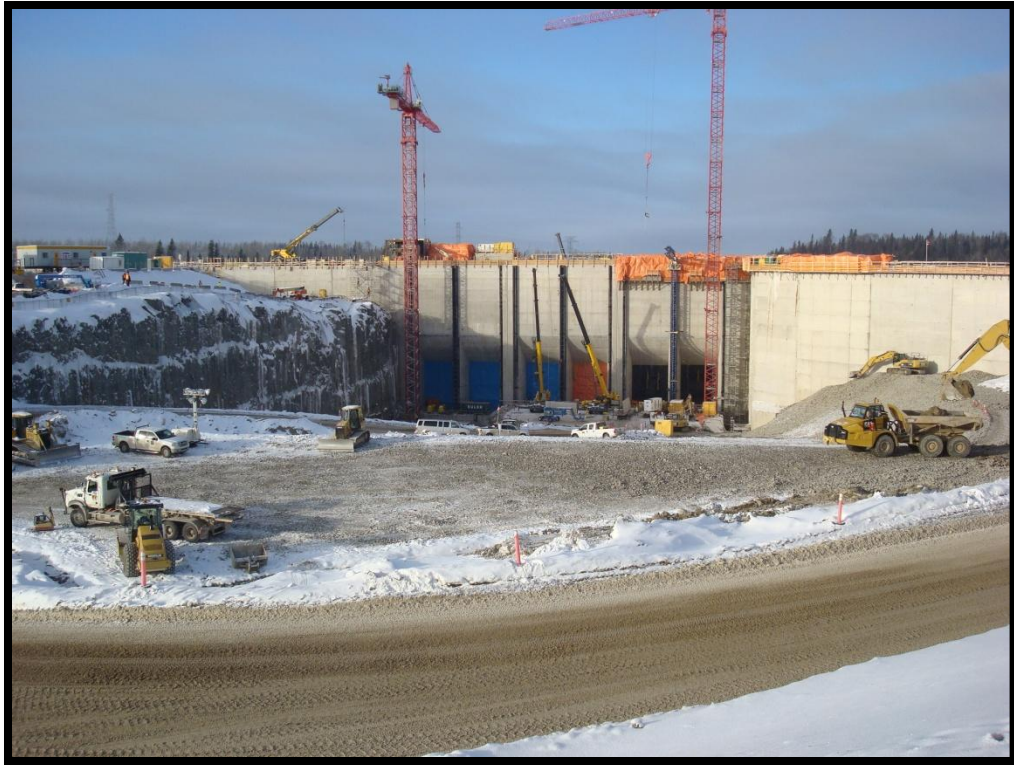
Figure 5: Smoky Falls Intake
