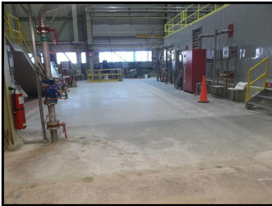
Figure 1: Little Long - Result of grout injection on Generator Floor
