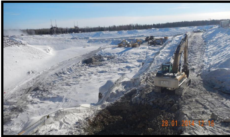
Figure 4: Smoky Falls excavating Intake Pad approach channel
