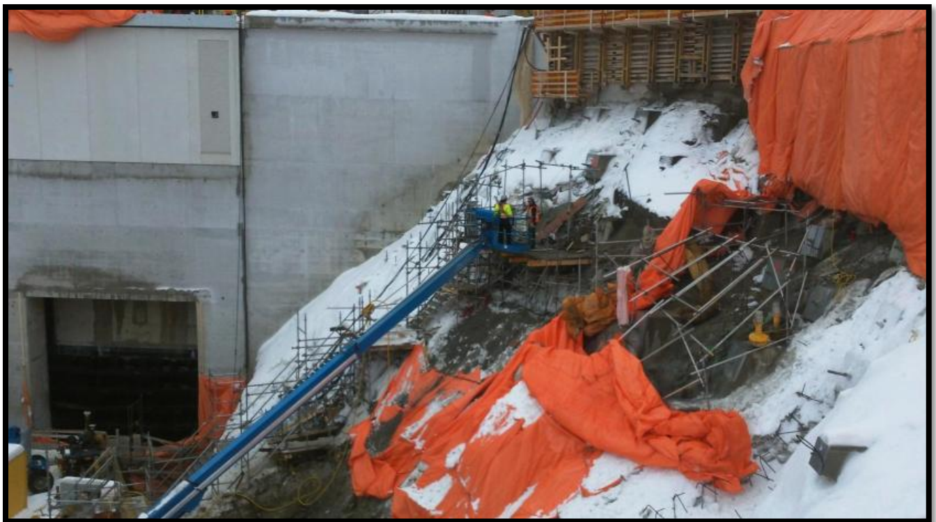
Figure 5: Zone 5 (west side wall) rebar installation
