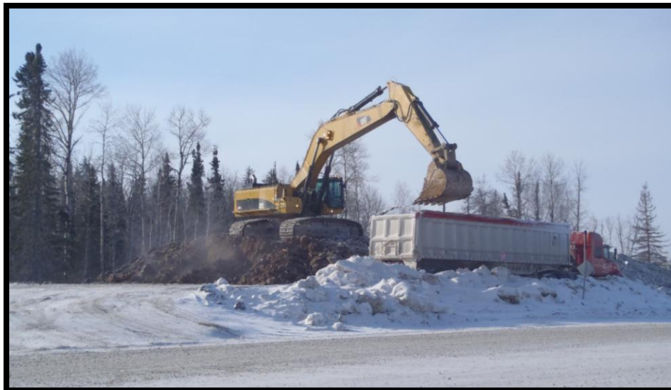
Figure 5: Removing the soil stockpiles at Smoky Falls
