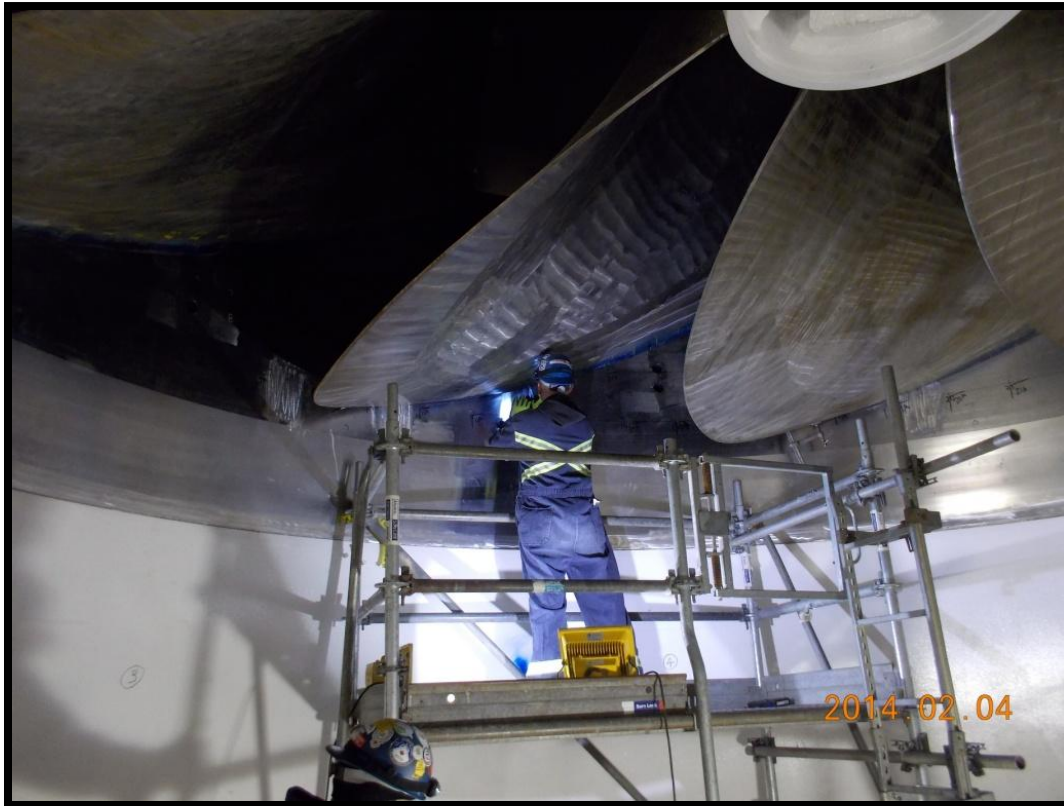
Figure 2: Harmon runner blade inspection
