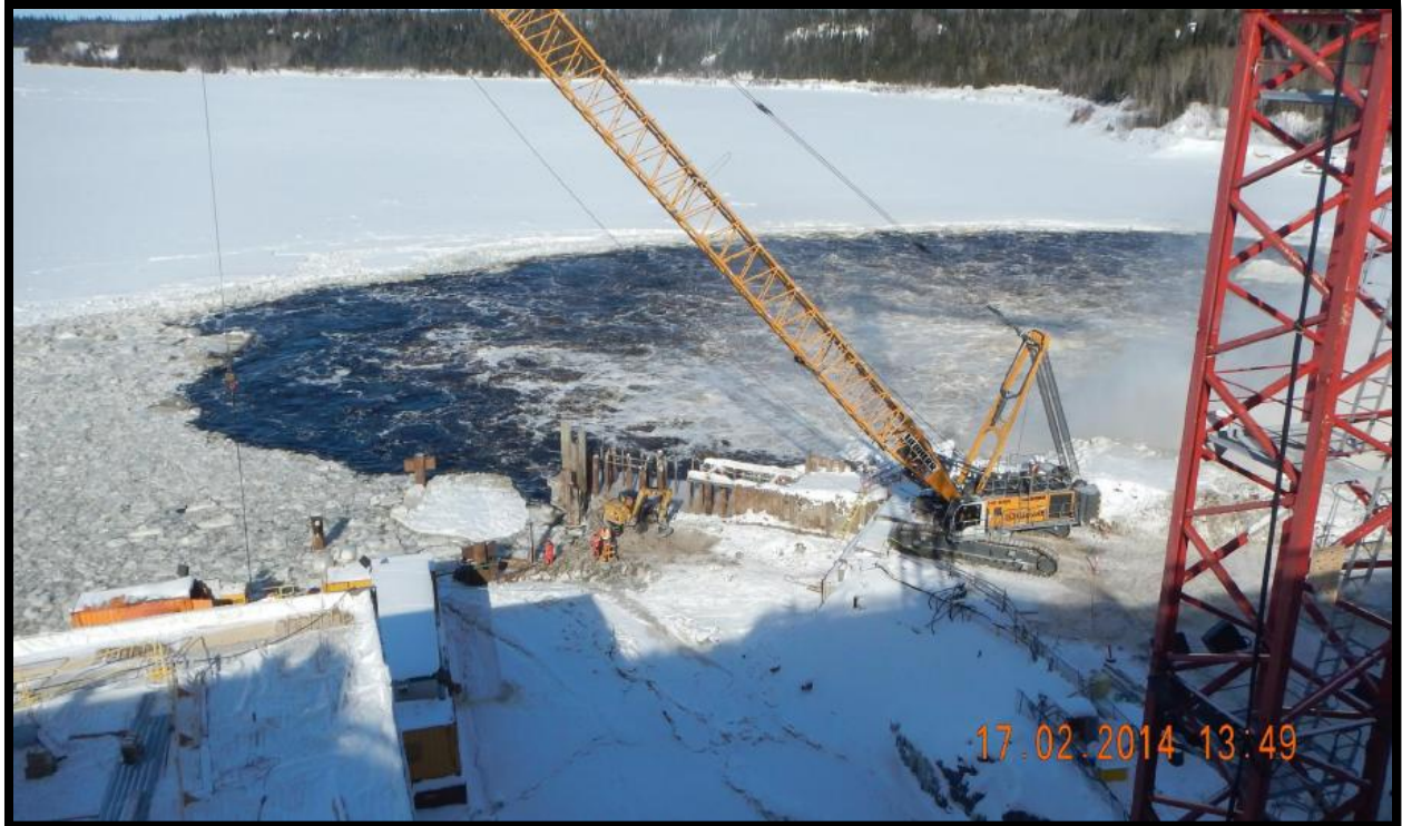
Figure 3: Kipling Cofferdam Removal
