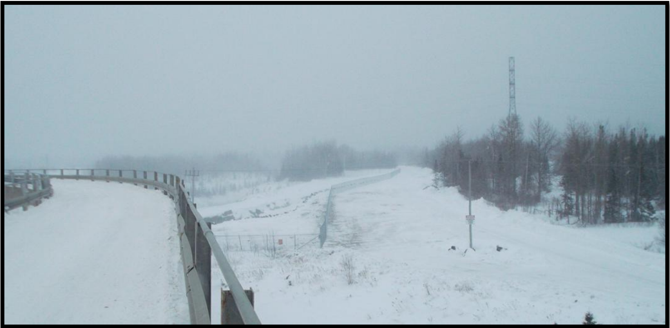
Figure 1: Little Long Permanent Fence
