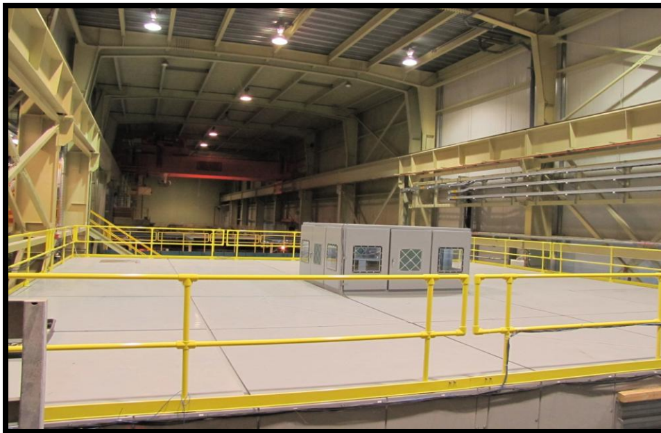
Figure 3: Kipling unit 3 inspections completed and Demonstration and Trial run in progress.
