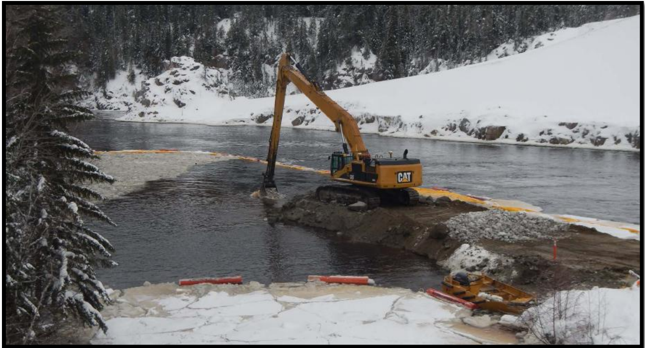
Figure 5: Smoky Falls fish habitat shoal construction (placing cobble)
