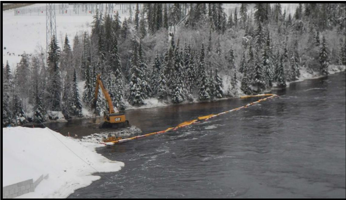
Figure 4: Smoky Falls Fish Habitat Shoal – Sediment contained by curtain
