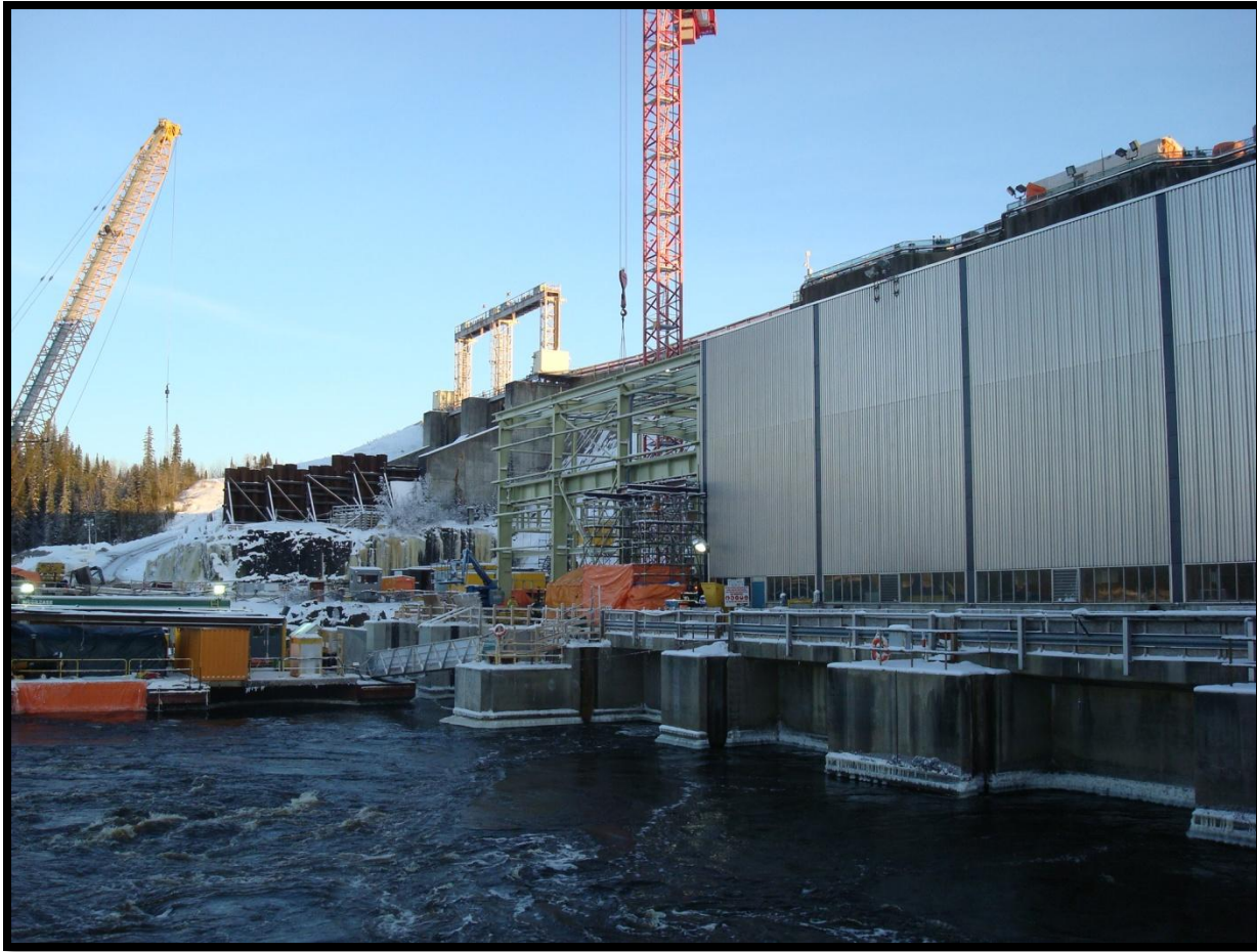
Figure 3: Kipling Superstructure erection
