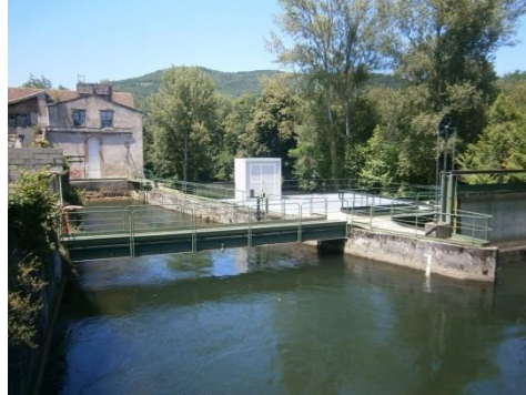
view on the power plant where first field tests on fish mortality were conducted in 2016
