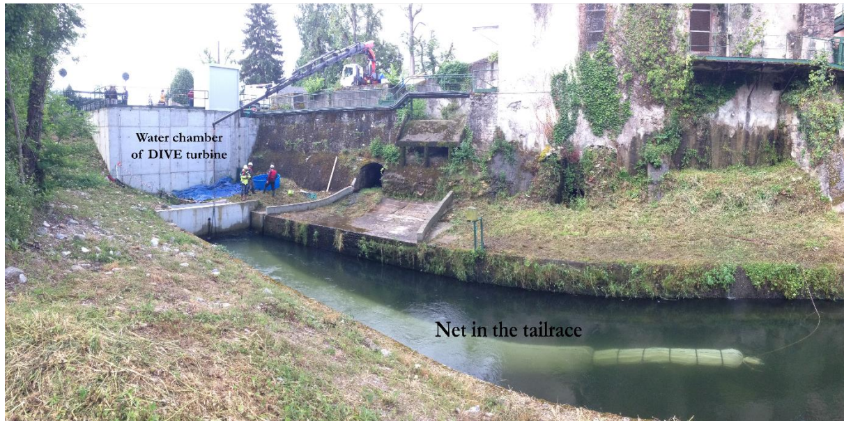
test facility during the test, view from downstream
