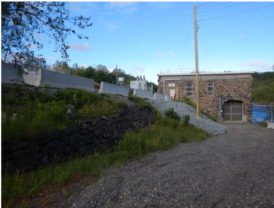
Figure 7: Service road running from between the two dam structures and the east entry to powerhouse.
