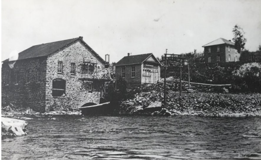
Figure 24: pre-1915, showing original powerhouse, transformer building and a staff residence on the hill. Source, OPG. Reproduced from Unterman McPhail (SCRR 2017).
