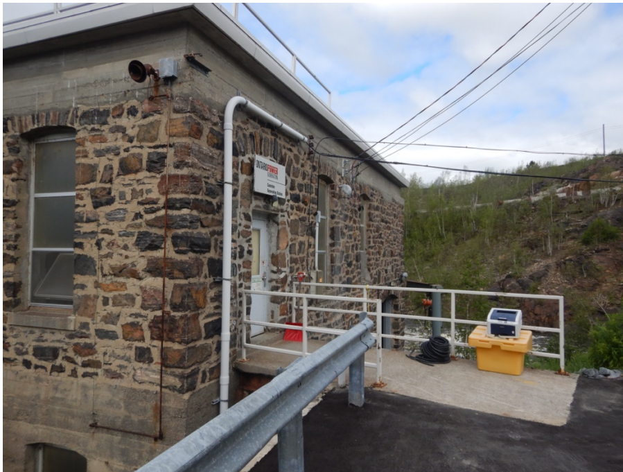
Figure 23: South and east walls
