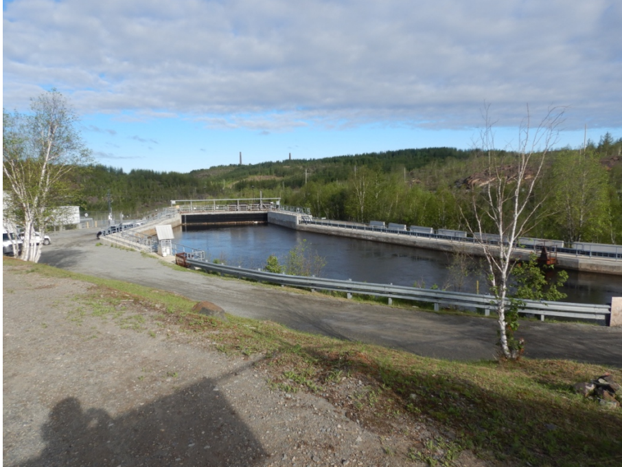
Figure 8: Forebay canal with headworks in distance. Note smelter chimneys on horizon.
