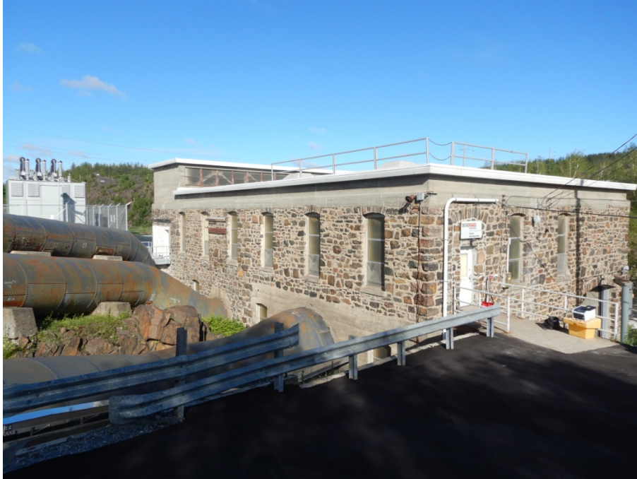
Figure 18: General view of east and south walls. Former transformer building / carpenter shed, now a transformer / switch facility in the upper left of photo.
