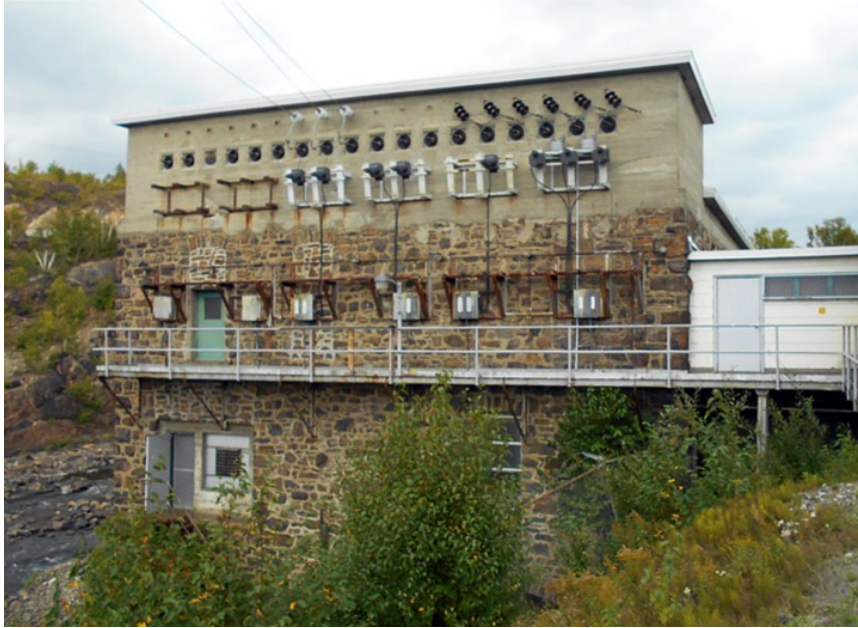
Figure 26: 2016 West wall of powerhouse. Reproduced from Unterman McPhail (SCRR 2017).
