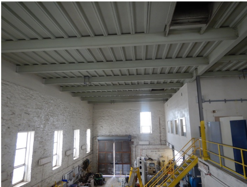
Figure 27: view of powerhouse interior showing ceiling form.
