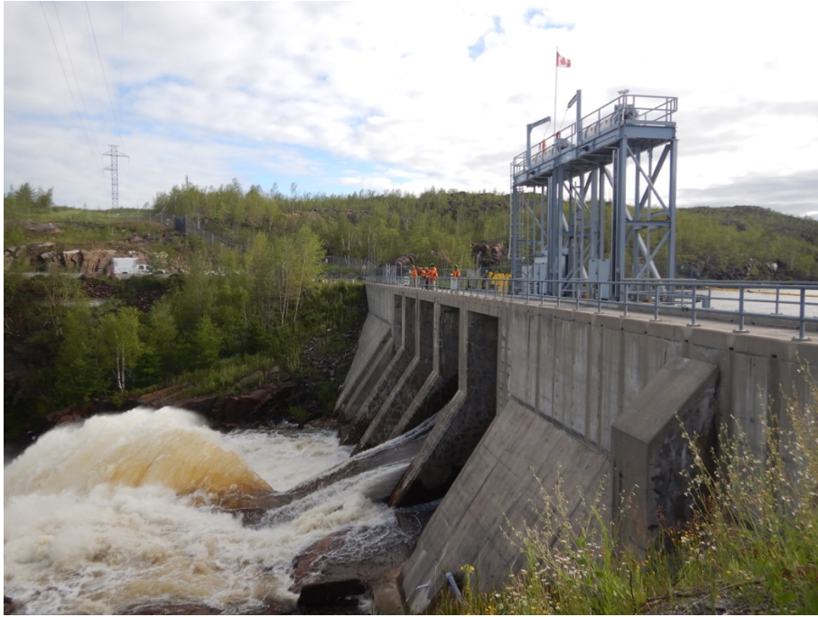
Figure 4: View of dam and sluiceways (2020).
