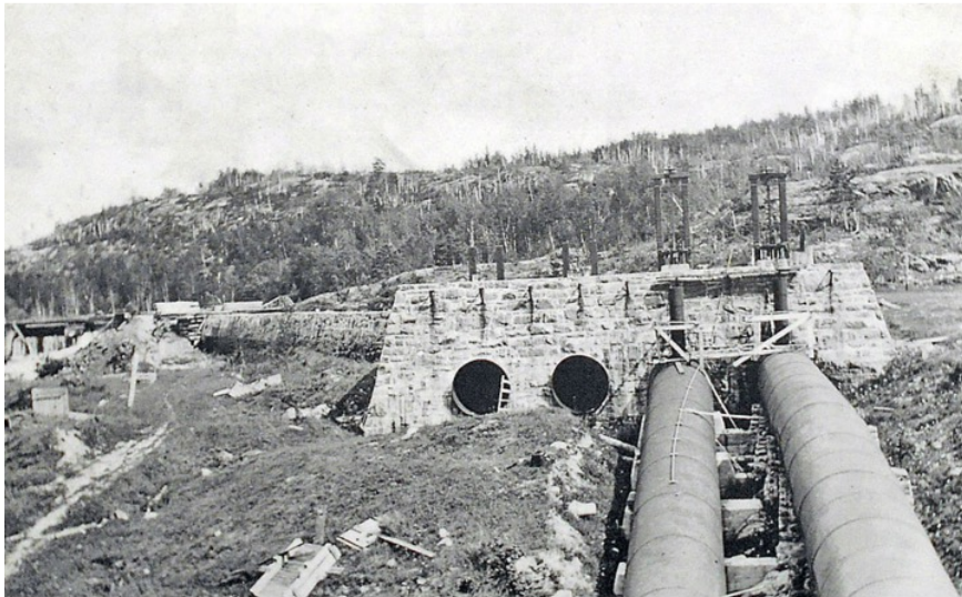
Figure 5: Headworks and penstocks 1 and 2 under construction. Dam visible to left of photo. Source, OPG. Reproduced from Unterman McPhail (SCRR 2017).
