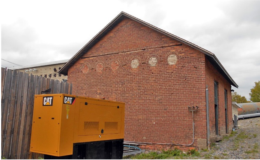
Figure 34: Former Transformer House, later Carpenter Shop, demolished between 2016 and 2022. Reproduced from Unterman McPhail (SCRR 2017).
