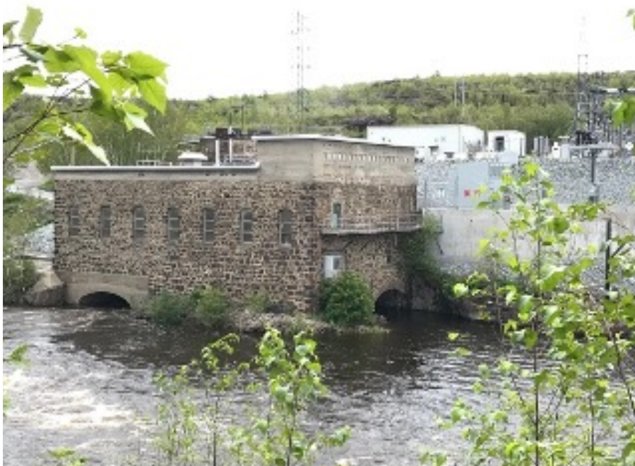
Figure 15: View of the powerhouse from the north bank of the Wanipetei River showing west and north faces and post-1954 roof. The 1915 extension can be discerned by the difference in stonework and mortar.
