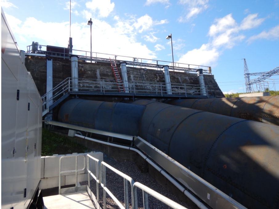
Figure 10: View of the headworks.
