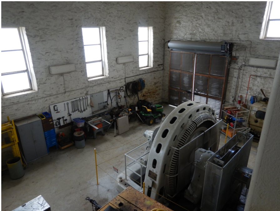
Figure 31: View from mezzanine. Unit G3 in foreground, service door to right.
