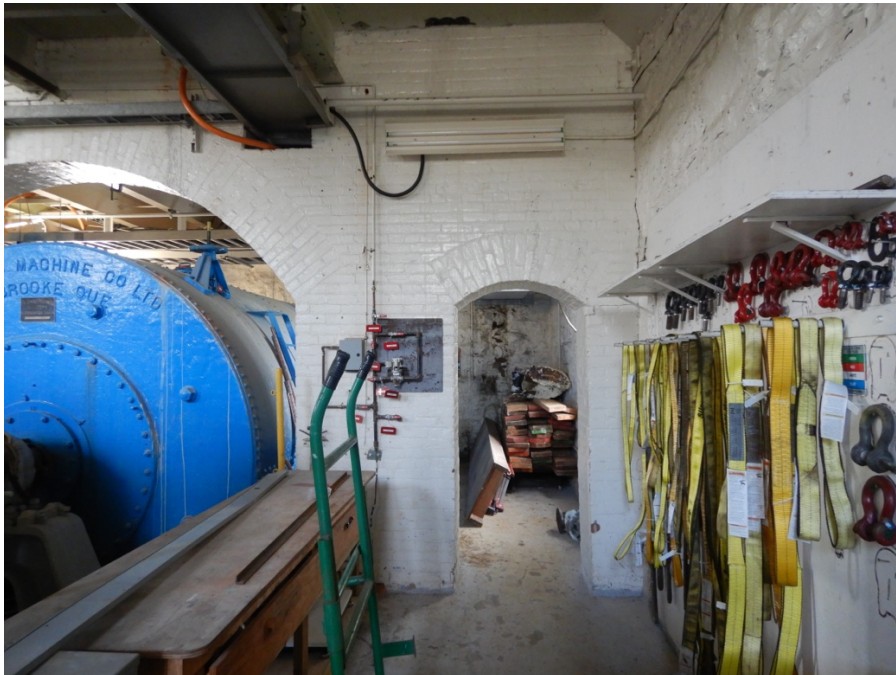
Figure 33: Powerhouse interior detail showing brick partition supporting mezzanine, brick arch above door, and Unit 1 turbine.
