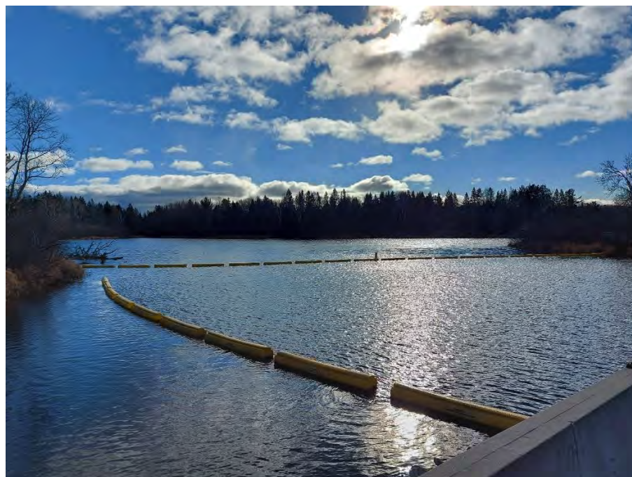
Figure 2-5 Forebay/Reservoir and Boom Lines
