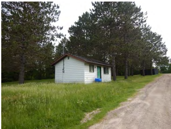
Figure 13: Bingham Chute GS, office / lunchroom.
