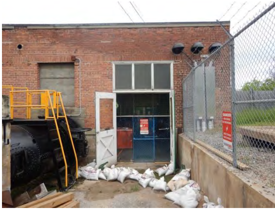
Figure 6: Bingham Chute GS, view of powerhouse, south wall entry door.
