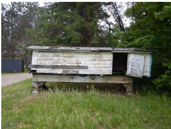
Figure 14: Bingham Chute GS, log lifting crane.
