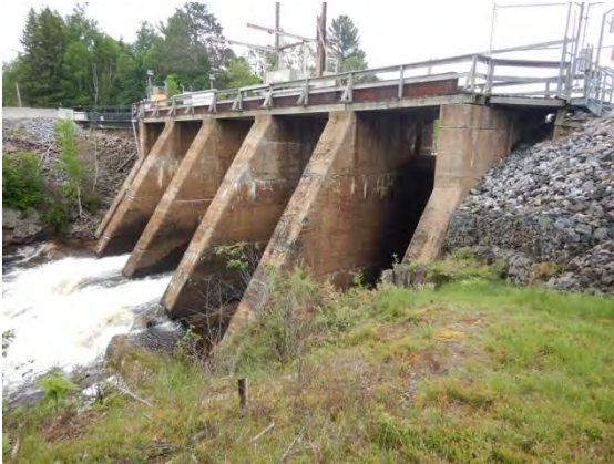
Figure 5: View east of the dam on the South River.
