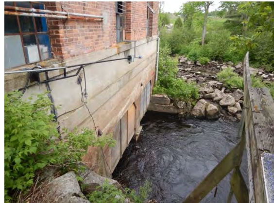
Figure 10: View west showing tailrace exit from powerhouse.
