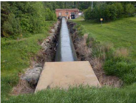
Figure 7: View north of penstock and powerhouse. Compare with Figure 15.
