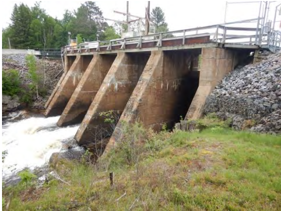
Figure 1: Bingham Chute GS, main dam.
