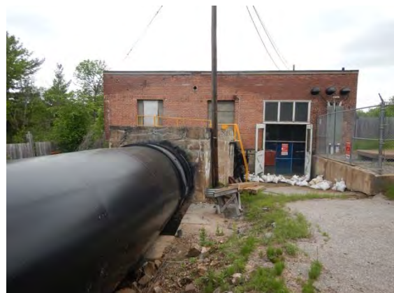
Figure 4: Bingham Chute GS, view of powerhouse.
