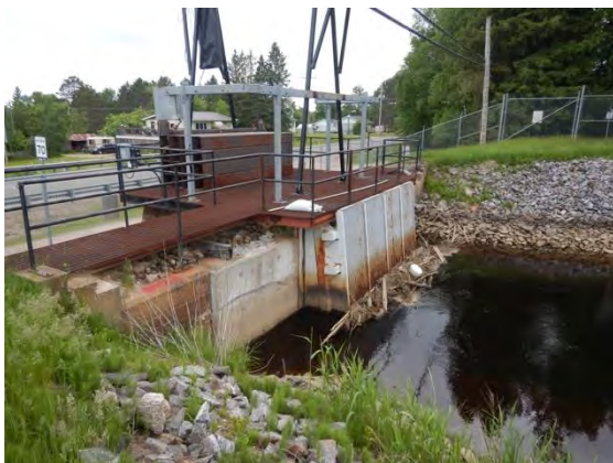
Figure 2: Bingham Chute GS, intake, headworks.
