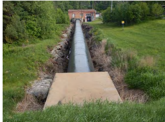
Figure 3: Bingham Chute GS, penstock.
