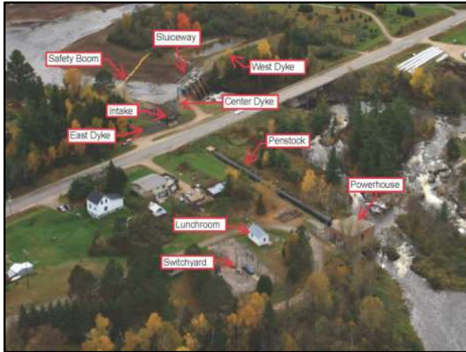
Photograph 1. Oblique Aerial View of Powerhouse and Associated Structures (from Tetra Tech Life Extension Report)
