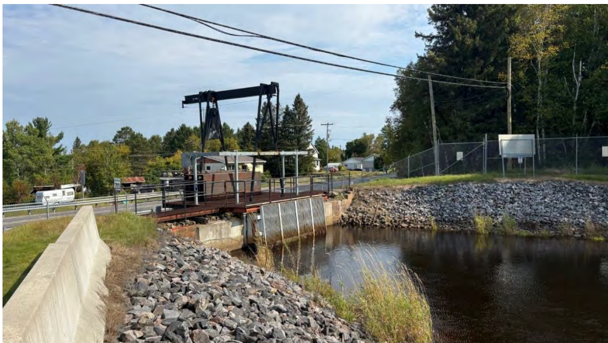
Figure 2-3 Intake and Trashrack
