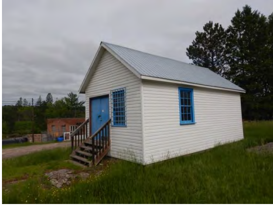
Figure 12: Bingham Chute GS, storage building.
