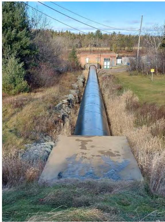
Figure 2-6 Penstock and Powerhouse
