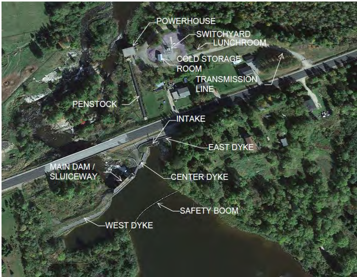
Figure 2-1 Aerial View of Powerhouse and Associated Structures (Tetra Tech, 2022, Google aerial image)
