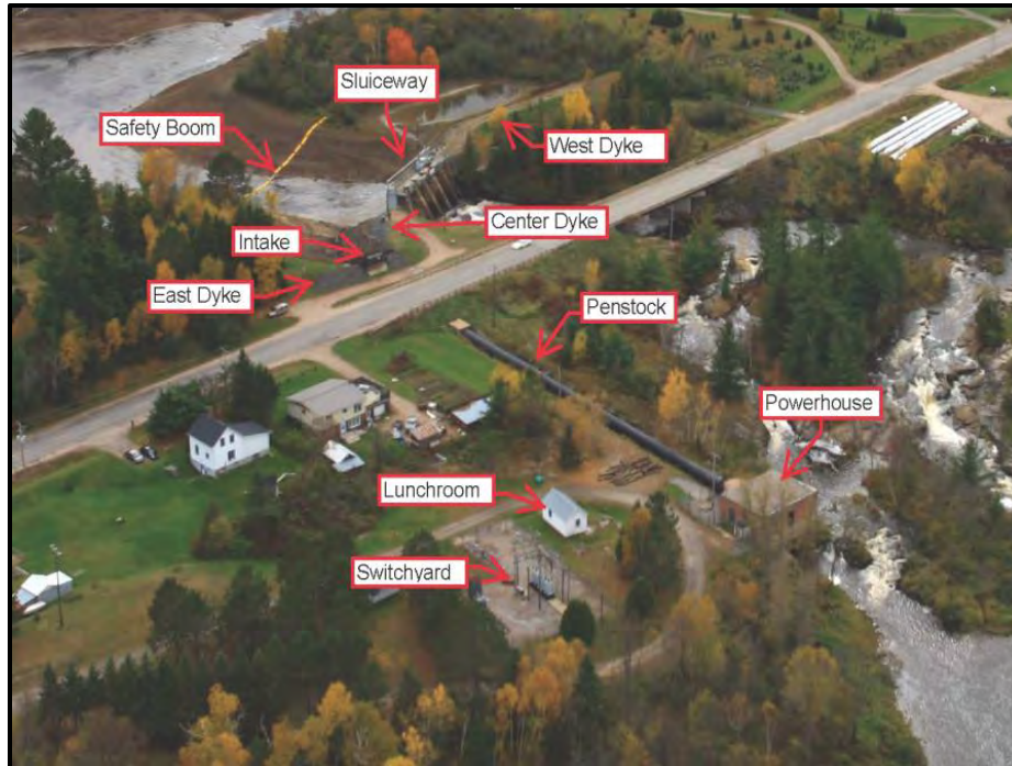
Photograph 1. Oblique Aerial View of Powerhouse and Associated Structures (from Tetra Tech Life Extension Report)
