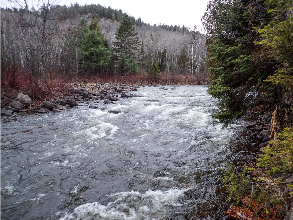
Figure 3-5. View of the spillway, looking upstream from the farthest upstream location examined for spawning Lake Whitefish. November 15, 2022.
